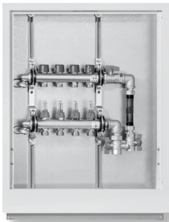
Fig.: Connection on the right
