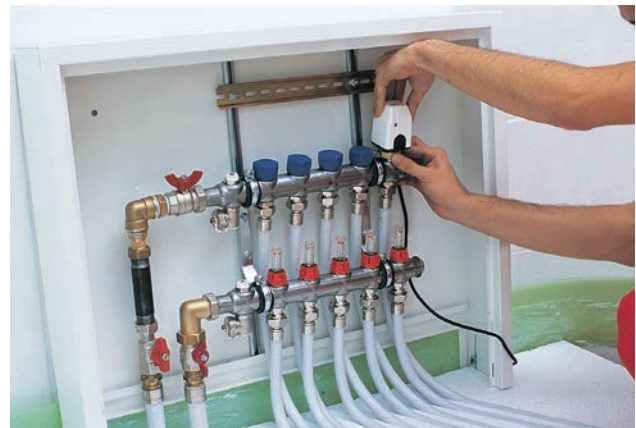
Setting of PRINETO actuators
