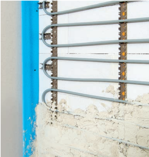
Installing PRINETO wall heating wet
